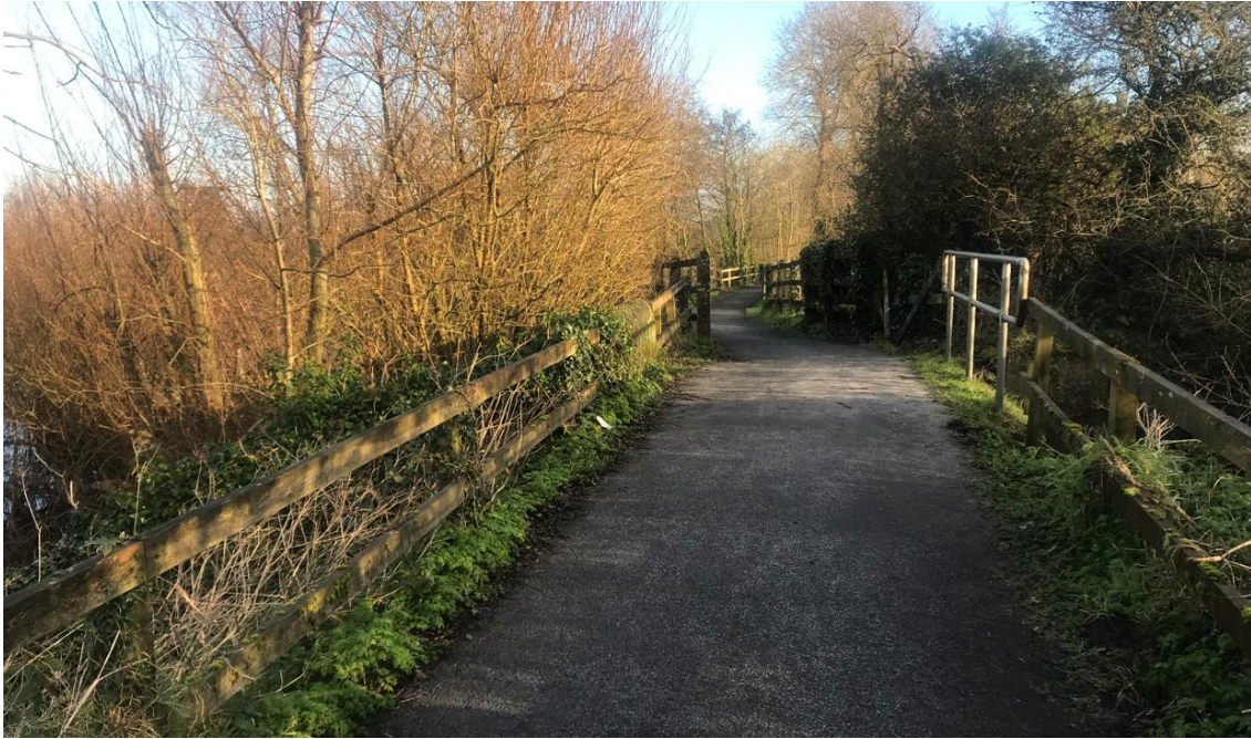
Figure 3-10: Existing Bridge No 1
