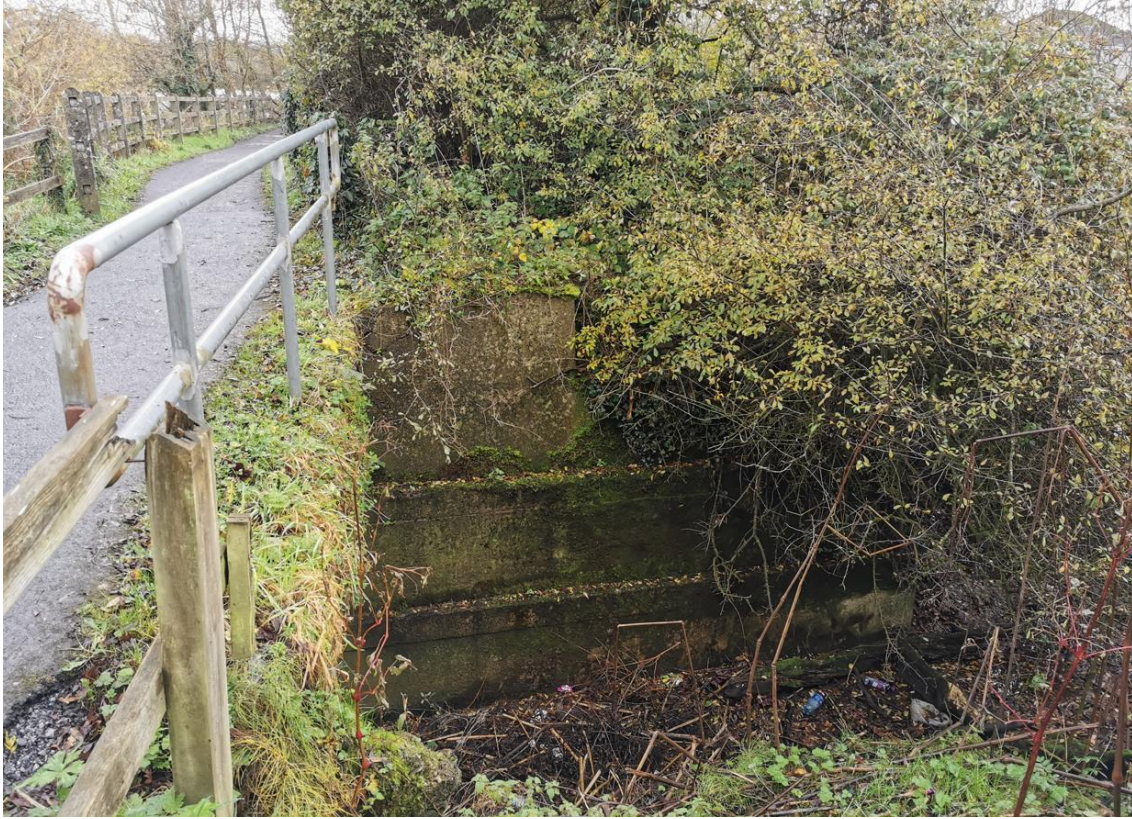
Figure 3-12: Existing abutment wall (proposed to be decommissioned)
