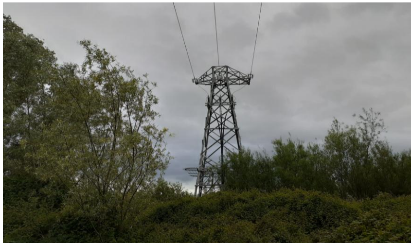
Figure 3-61: Overhead ESB utilities
