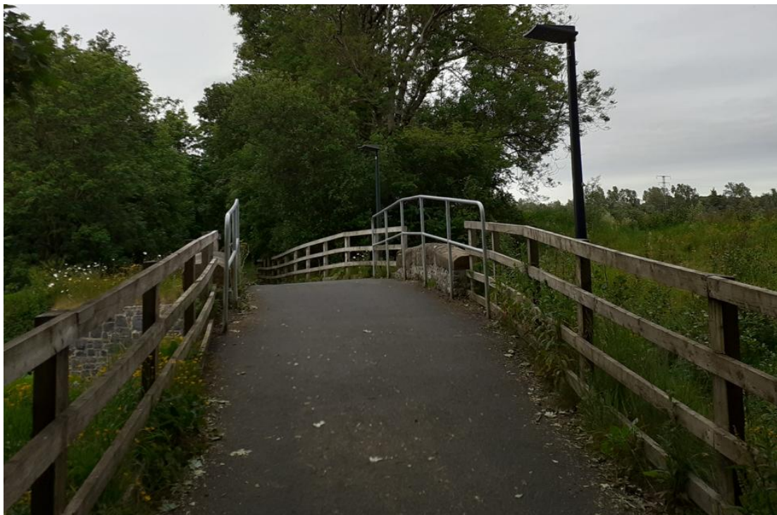
Figure 3-3: Existing bridge at CH400
