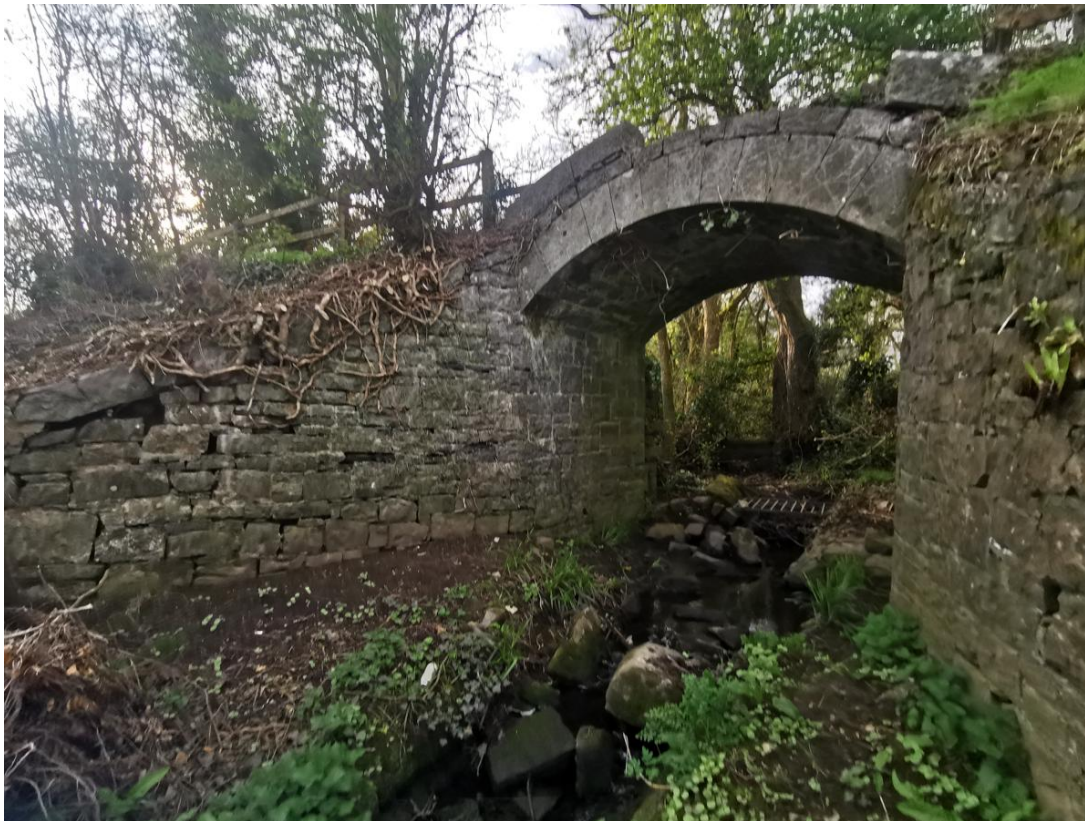
Figure 3-17: View of Bridge 2 from bank of drain
