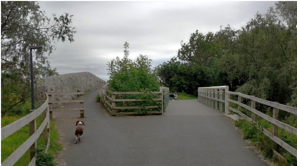
Figure 3-1: Existing Bridge at River Groody
