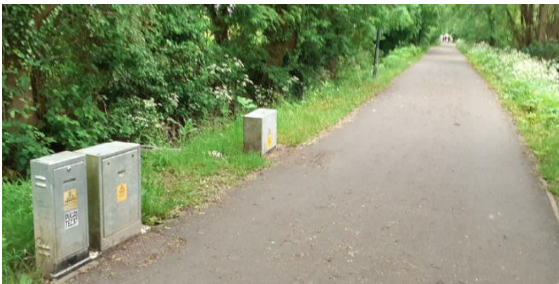
Figure 3-4: Existing path to be resurfaced
