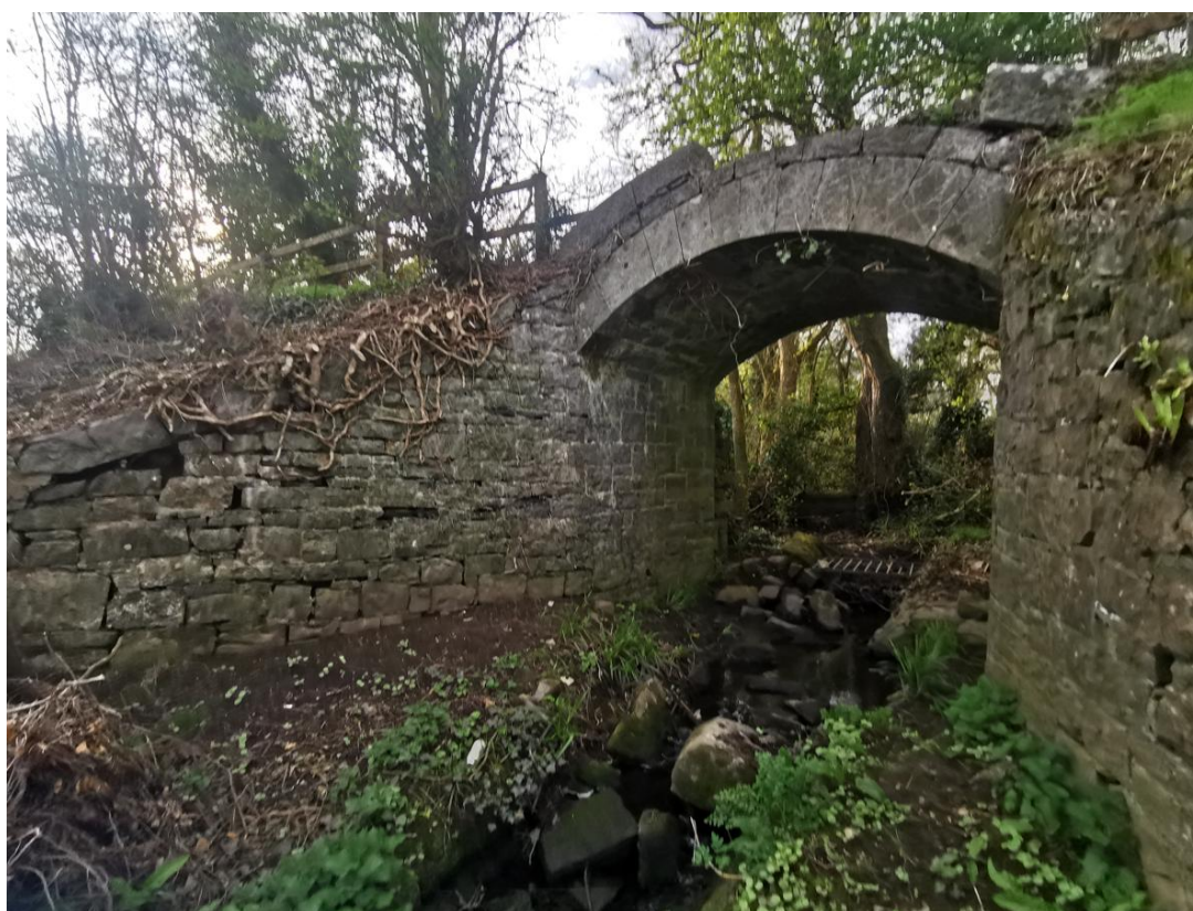
Figure 3-17: View of Bridge 2 from bank of drain
