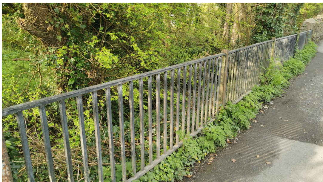
Figure 3-19: : Existing railing between Bridge 2 and Bridge 3
