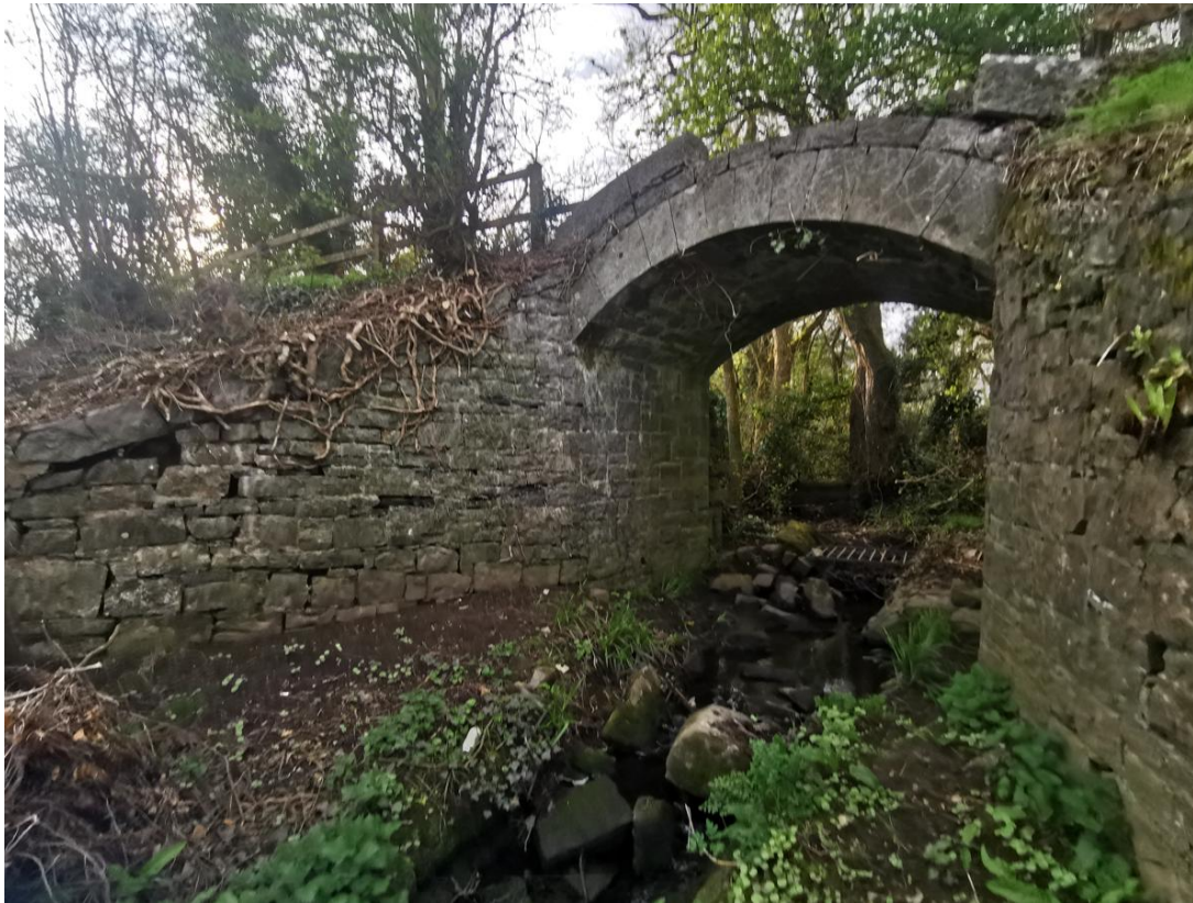
Figure 3-17: View of Bridge 2 from bank of drain
