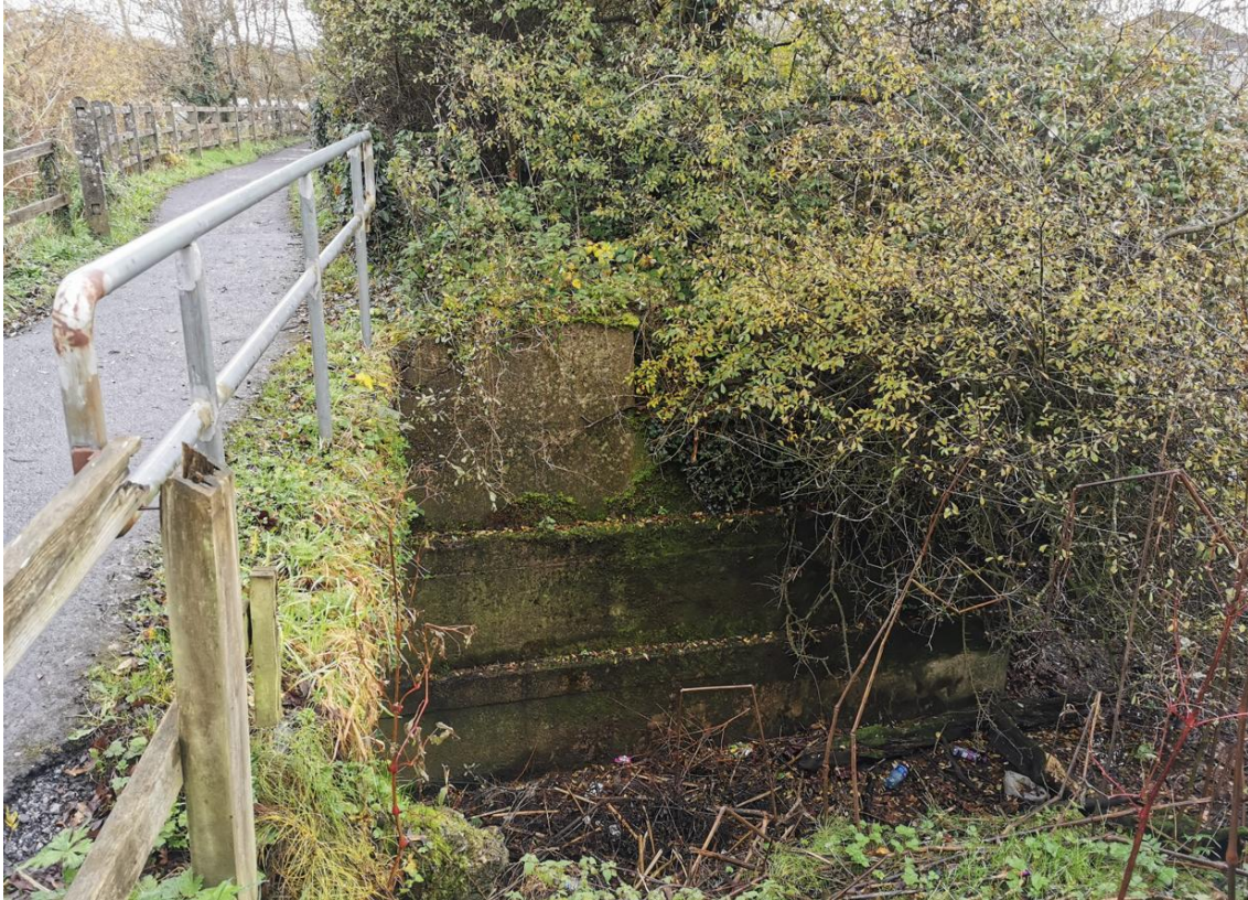
Figure 3-12: Existing abutment wall (proposed to be decommissioned)
