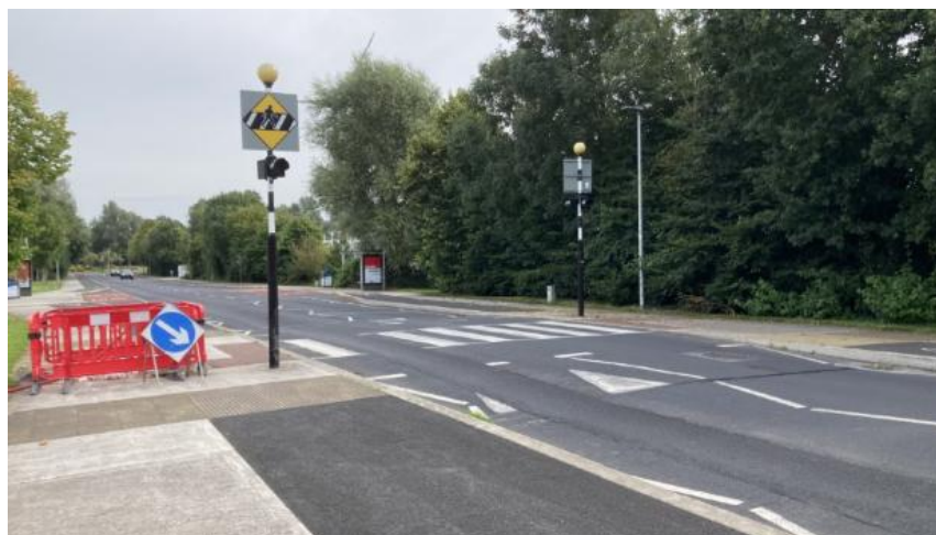
Figure 3-67: Existing Zebra crossing on Plassey Park Road
