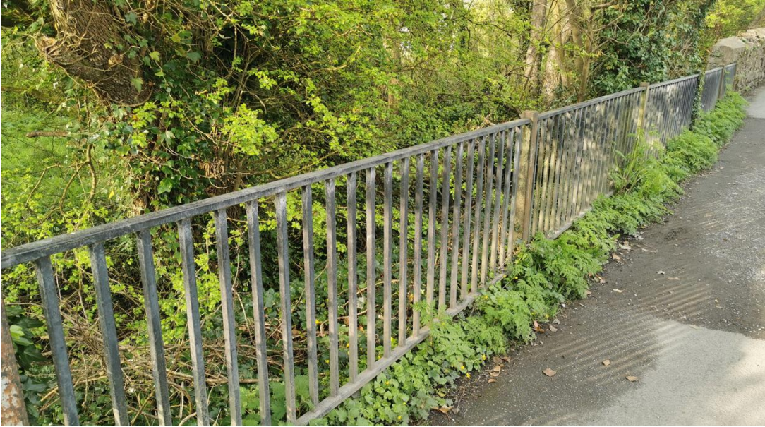
Figure 3-19: : Existing railing between Bridge 2 and Bridge 3
