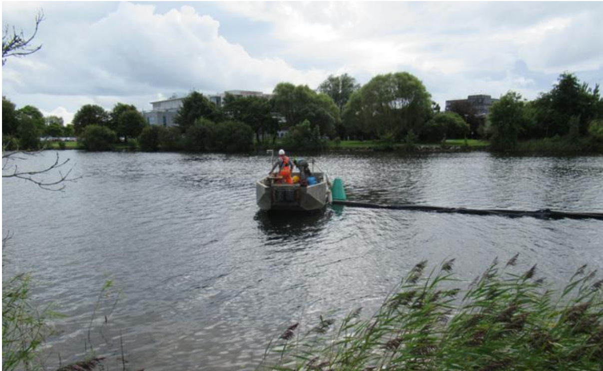
Figure 3-85: Installation of a silt curtain in the River Corrib, Co. Galway
