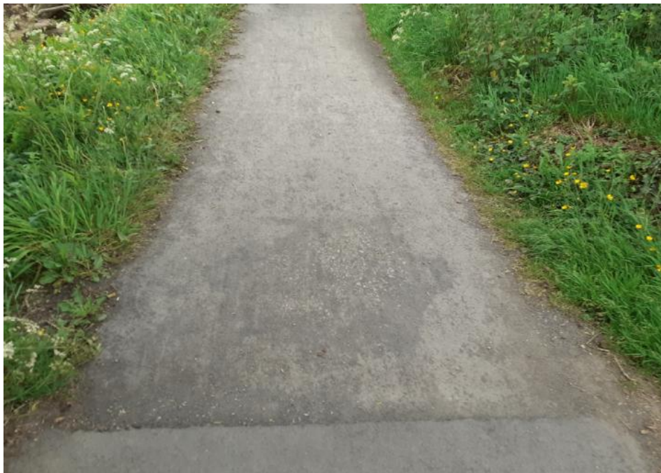
Figure 3-9: Path surface changes from paved to gravel and narrows to approximately 1.5m width
