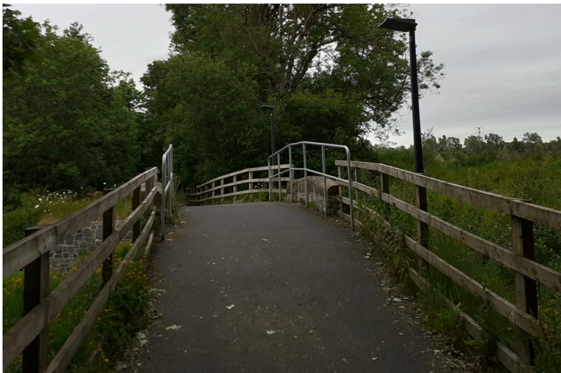
Figure 3-3: Existing bridge at CH400
