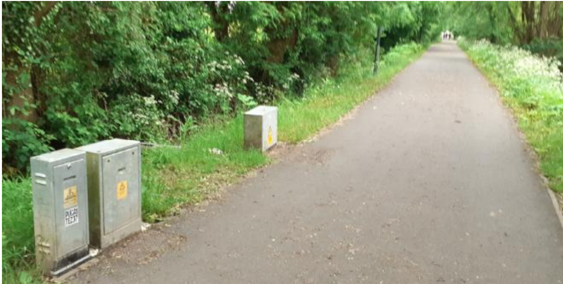
Figure 3-4: Existing path to be resurfaced
