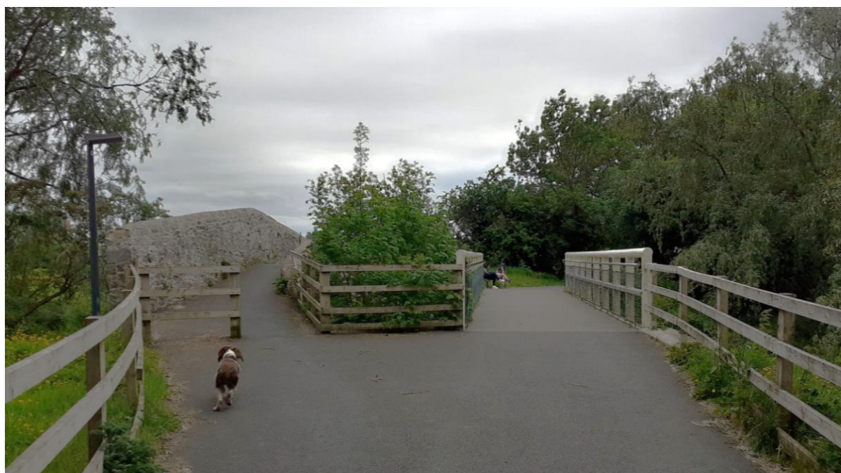
Figure 3-1: Existing Bridge at River Groody
