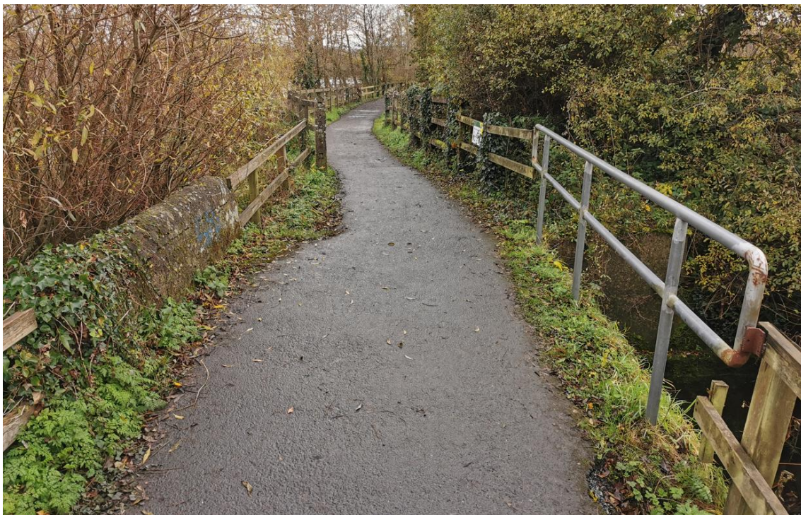
Figure 3-11: Existing bridge over land drain (Bridge 1)
