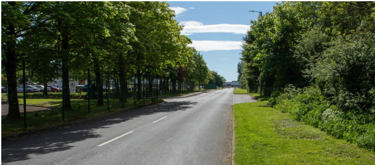
Figure 3-71: University Road (looking south)
