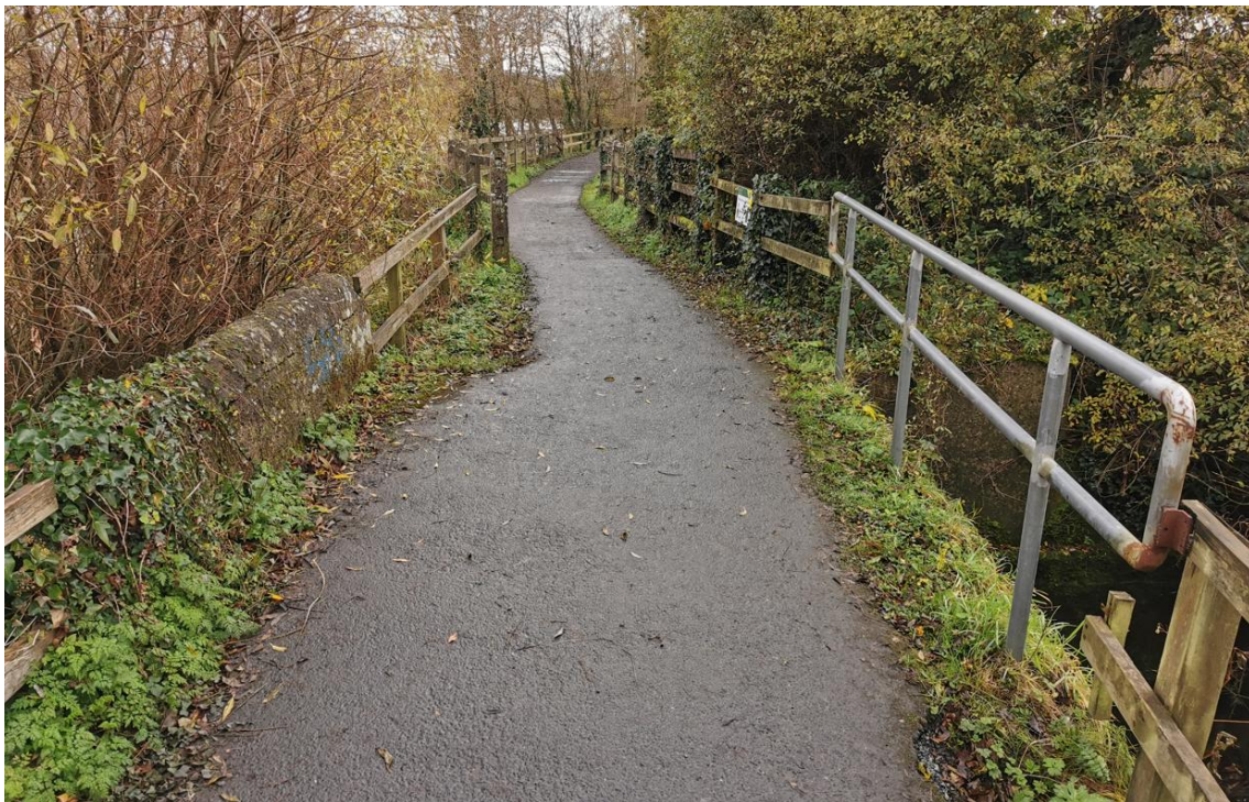
Figure 3-11: Existing bridge over land drain (Bridge 1)
