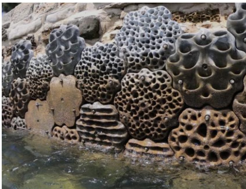
Figure 3-92: Example of aquatic plates to be installed on bridge abutments
