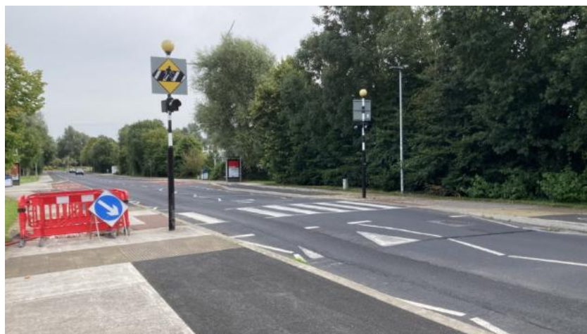
Figure 3-67: Existing Zebra crossing on Plassey Park Road
