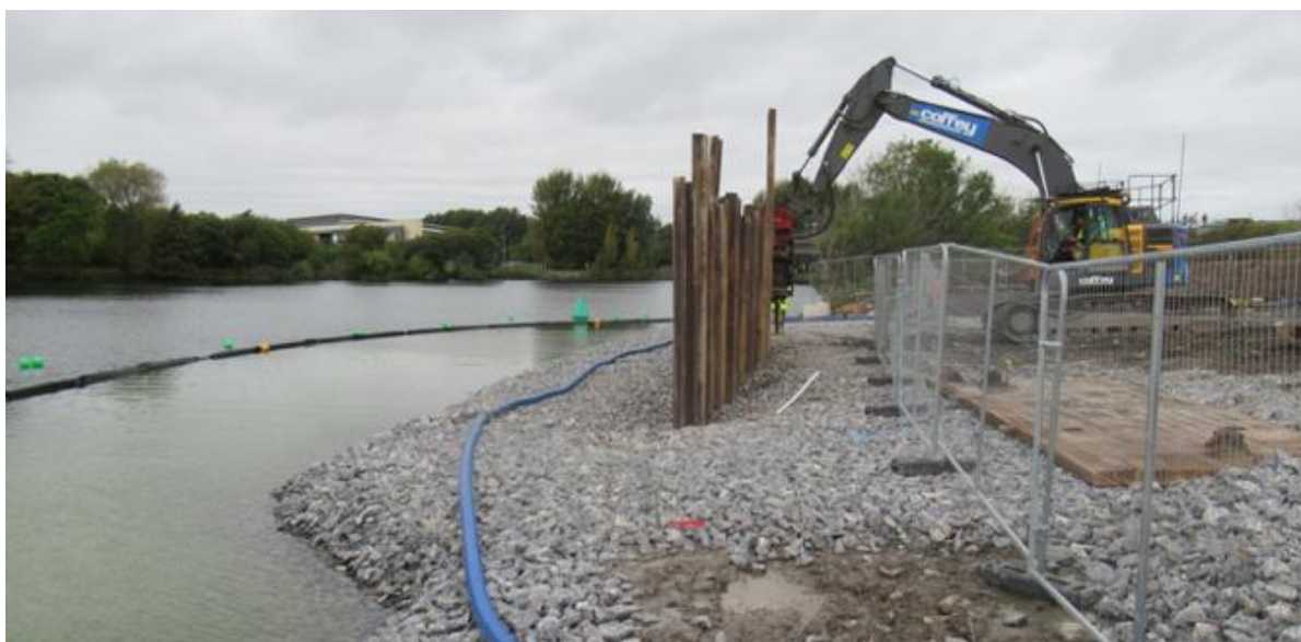
Figure 3-87: Example of sheet piling along the bank of the River Corrib
