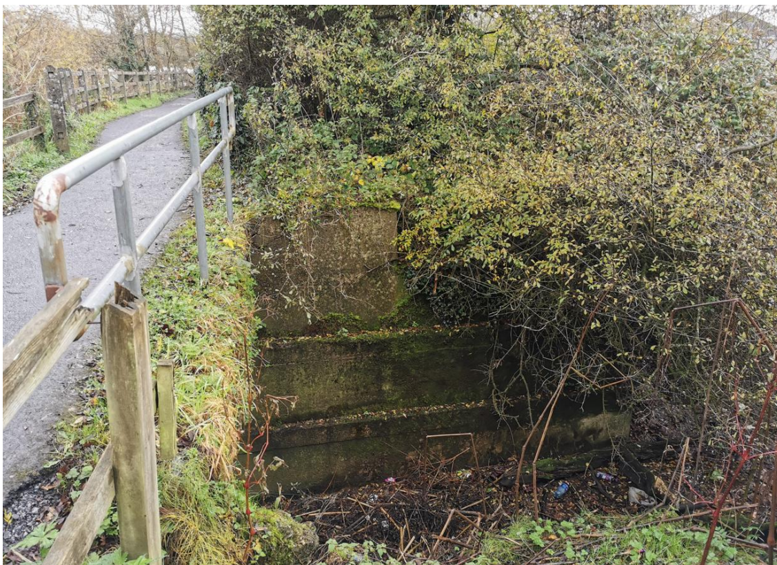
Figure 3-12: Existing abutment wall (proposed to be decommissioned)
