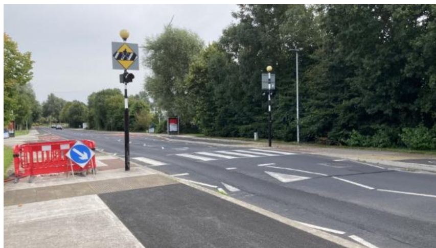
Figure 3-67: Existing Zebra crossing on Plassey Park Road
