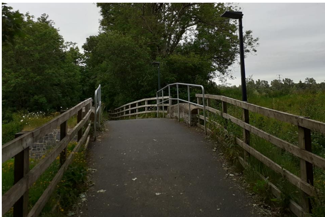
Figure 3-3: Existing bridge at CH400
