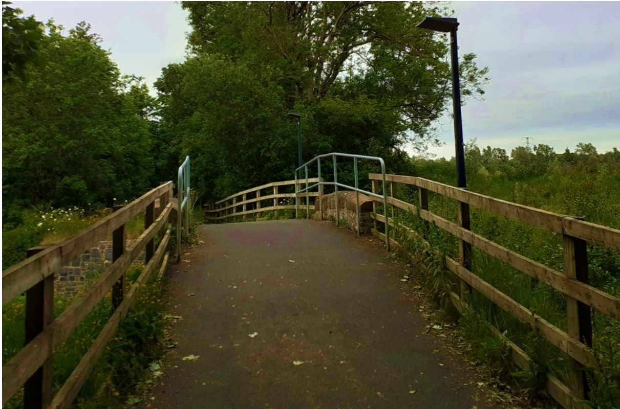
Figure 3-78: Existing bridge at CH400
