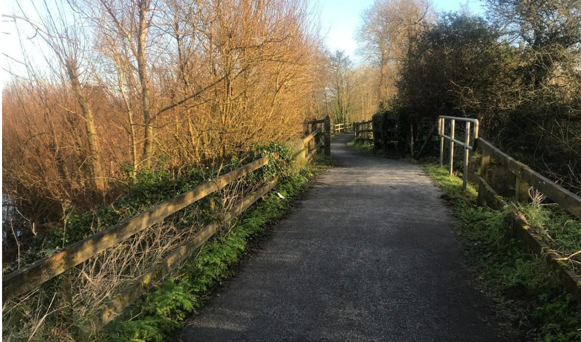
Figure 3-10: Existing Bridge No 1
