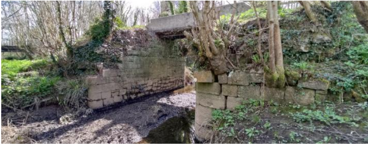
Figure 3-21: Shallow water level in Plassey Mill Race and existing abutments of Bridge 3
