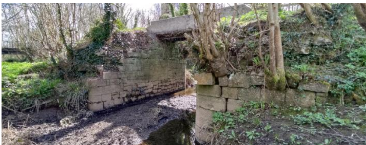
Figure 3-21: Shallow water level in Plassey Mill Race and existing abutments of Bridge 3
