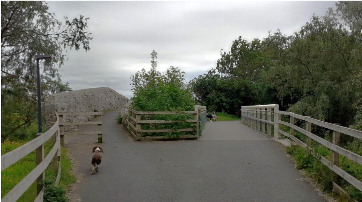
Figure 3-1: Existing Bridge at River Groody
