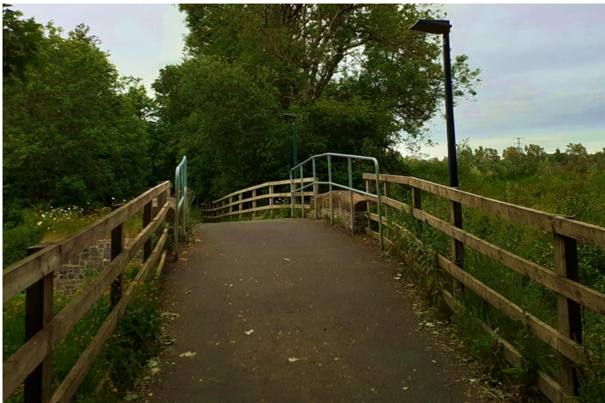
Figure 3-78: Existing bridge at CH400
