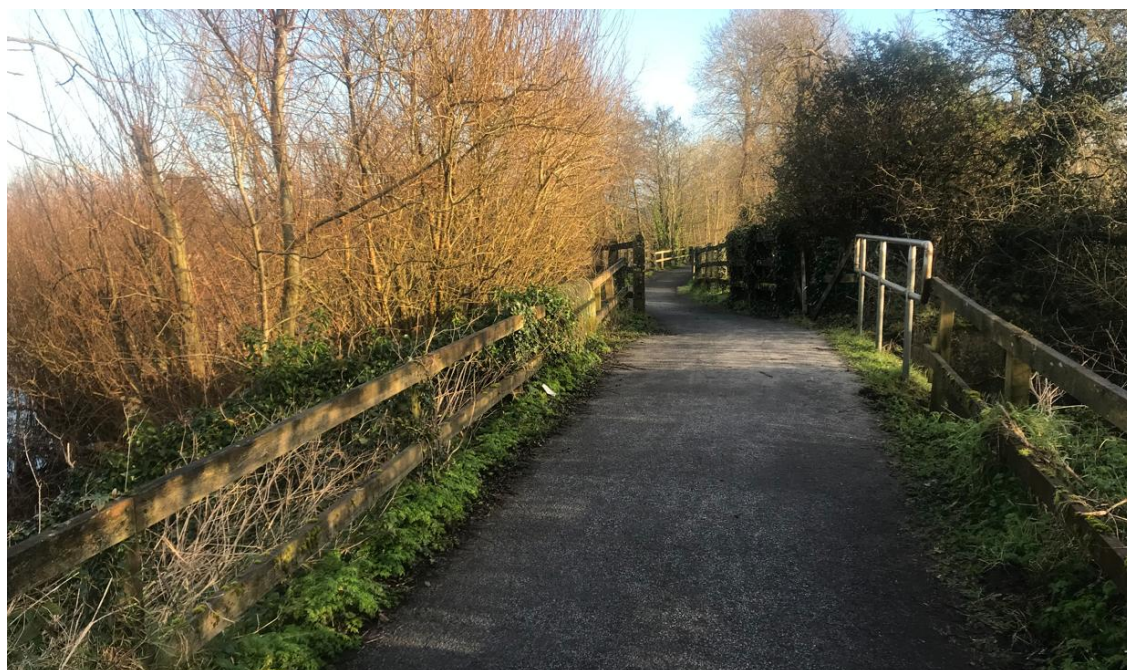
Figure 3-10: Existing Bridge No 1
